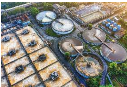
Waste Water Treatment Systems
